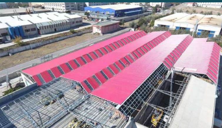
SANDWICH PANELS OR STEEL SHEET ROOF COVERS
