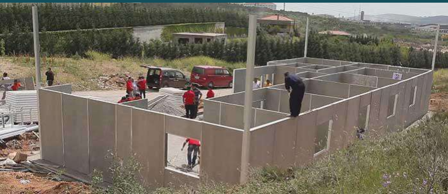
PREFABRICATED HOUSE ASSEMBLY
